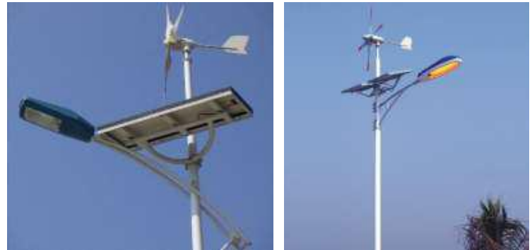
Figure 6. Solar Wind Hybrid Street Lights outdoors.
